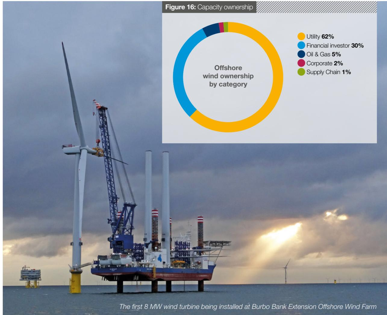
The first 8 MW wind turbine being installed at Burbo Bank Extension Offshore Wind Farm
