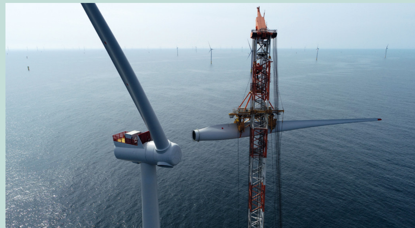
Construction works at Hornsea 1 offshore wind farm (Ørsted)
