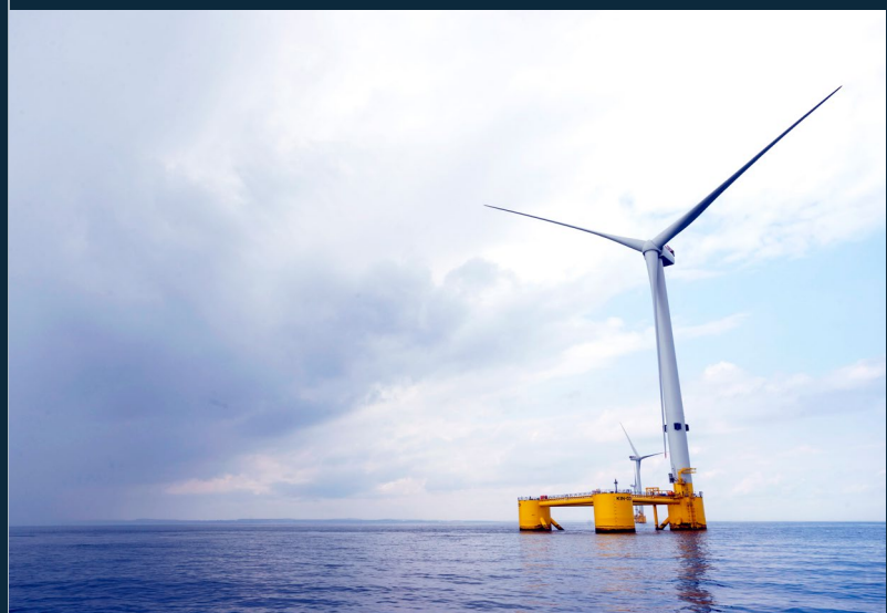
Image credit: Floating offshore wind farm, Flotation Energy
